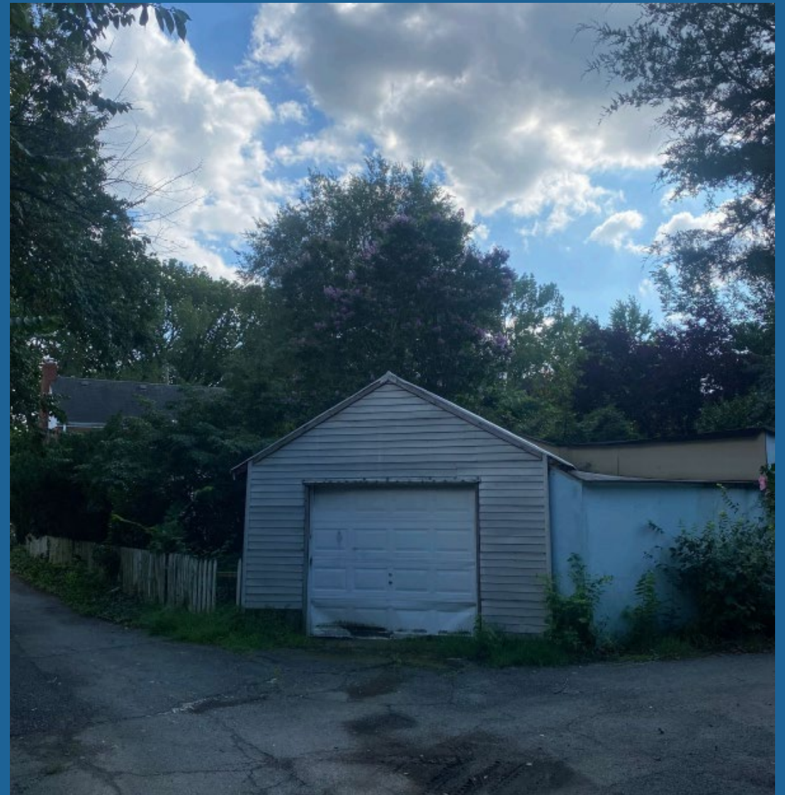
View of existing Alten garage looking south-southwest
